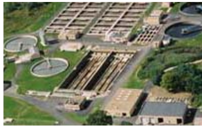
Bucklin Point WWTF
