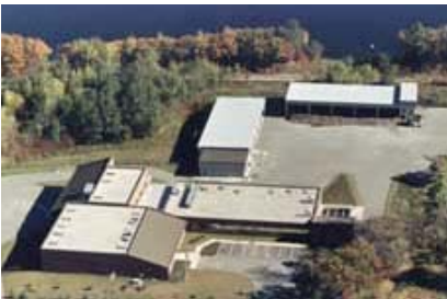
Gardiner Sanitary District Treatment Plant, Gardiner, ME
